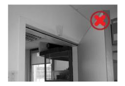
✓ Make sure to leave the area between the sensor and the ground clear and not obstructed by the door frame notably
